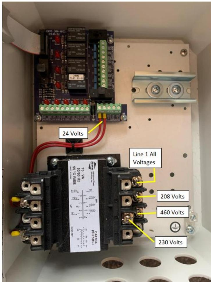
**Figure 4-7: Input Wiring**
