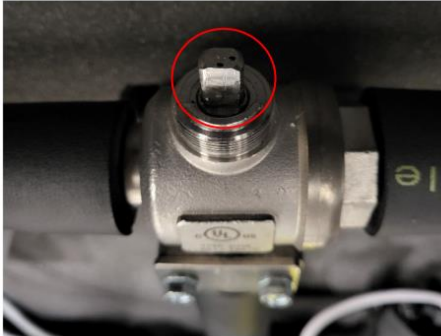
Disabling HIT Valve Visual Check
