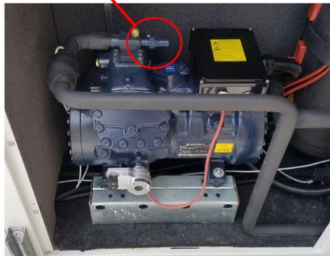
Discharge Service Valve Anatomy
