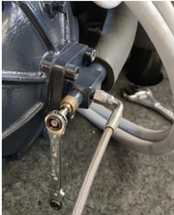
Charging the compressor w/ CO2 Refrigerant
