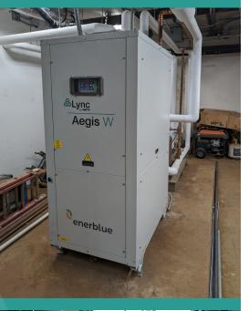
with the chiller water loop, which runs at a temperature of 50-55°F. This setup not only provided the necessary hot water for the resort but also contributed additional cooling to the chiller water loop, benefiting the cooling system of the hotel. This dual-purpose design leveraged the high efficiency of the Aegis heat pump, achieving a combined COP (Coefficient of Performance) of an impressive 6.4 by optimizing the energy used for both cooling and heating.
